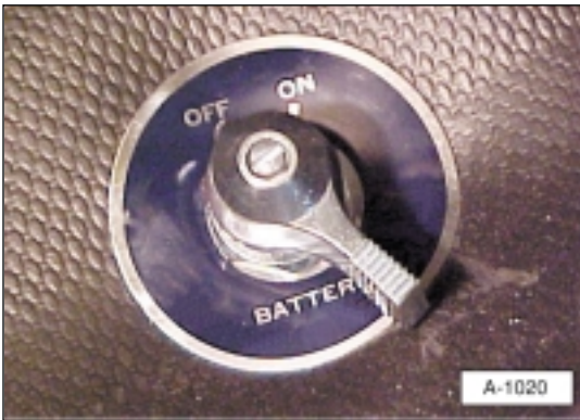
Illustration 7j. Cut-off switch mounted in cab of truck.
