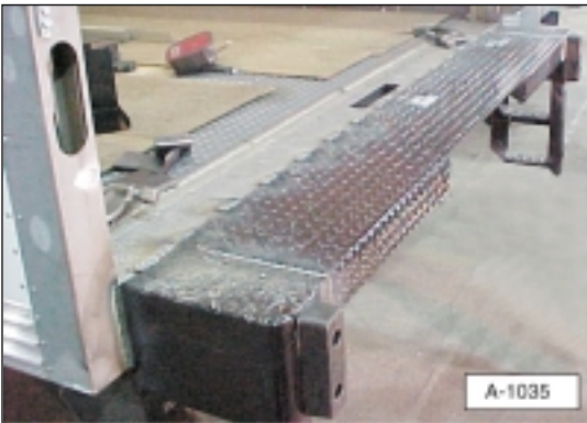
Illustration 17c. Correctly welded floor extension and dock bumper corners.
