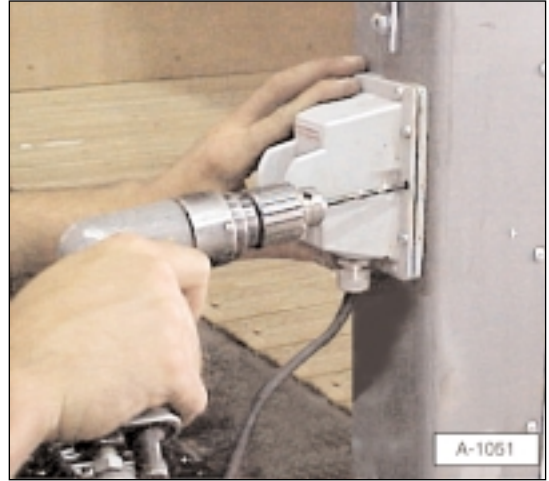
Illustration 16. Install the control switch.
