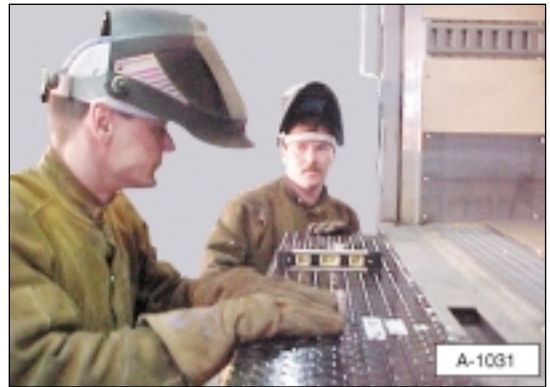
Illustration 4b. Level the floor extension.
